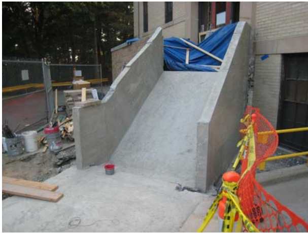
Newly poured concrete stairs
