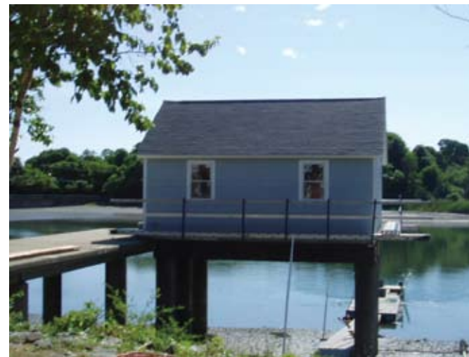
Auxiliary laboratory newly constructed on concrete pier above Smith Pool. FLUPSY is located at end of dock below building
