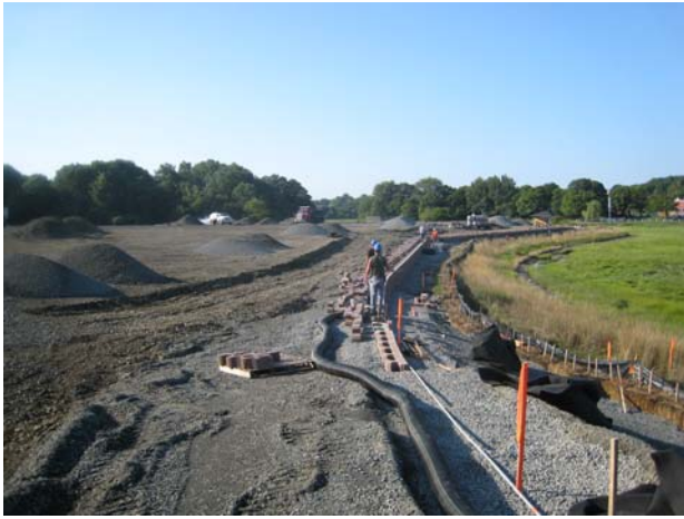
Construction of Retaining Wall
