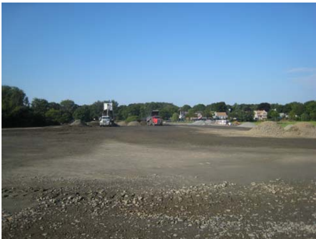
Delivery of Fill to Athletic Field Area
