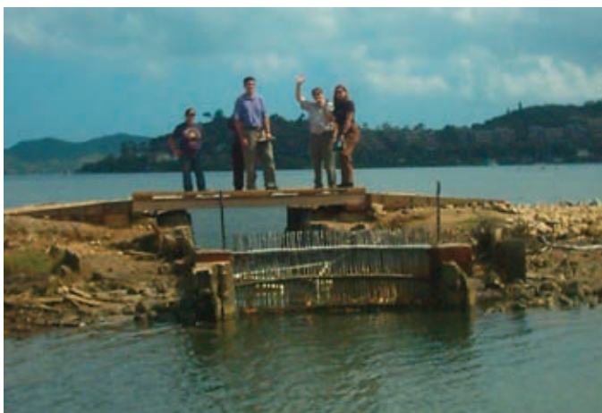
Fig. 14. Community members helped restore the mākāhā (fish gate) of He'eia fishpond. Mākāhā permit passage of water and small fish, but restrict escapement of larger fish. (Photo by J. Buttner)
