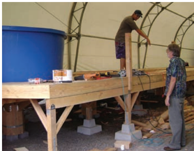
Fig. 8. Dr. Kevin Hopkins (right) consults with contractor assembling support for recirculating aquaculture systems being constructed at the UH Hilo new 5.0 ha aquaculture research/education/demonstration site. (Photo by J. Buttner)
